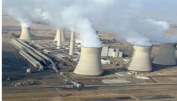
Figure. Thermal power plant
